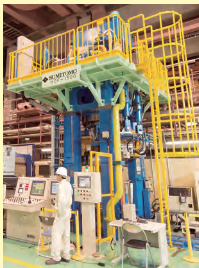
• Installation of Large-scale Forging Equipment
