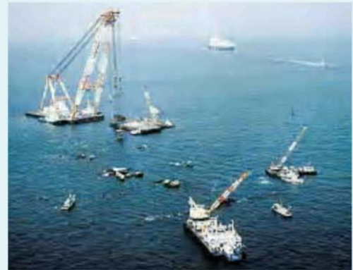
Fort No. 3 ("dai san kaiho") demolition
