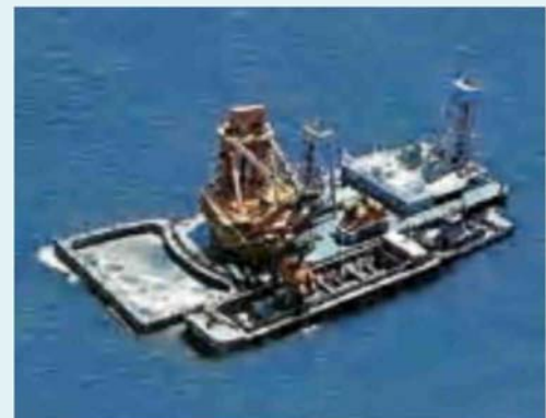
Nakayama Channel dredging conditions
