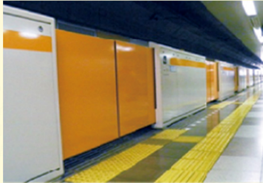
Platform screen doors (for fall prevention)
