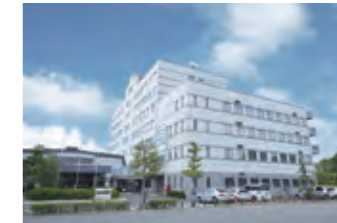
Fukuoka Incubation Center It has a total floor area of 1,365㎡ and consists of 17rooms.
