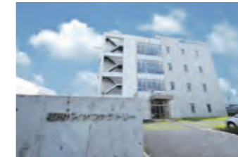
Fukuoka Biofactory It has a total floor area of 2,219㎡ and consists of 15rooms.
