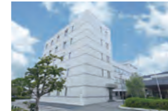
Fukuoka Bioinnovation Center It has a total floor area of 1,758㎡ and consists of 12rooms.
