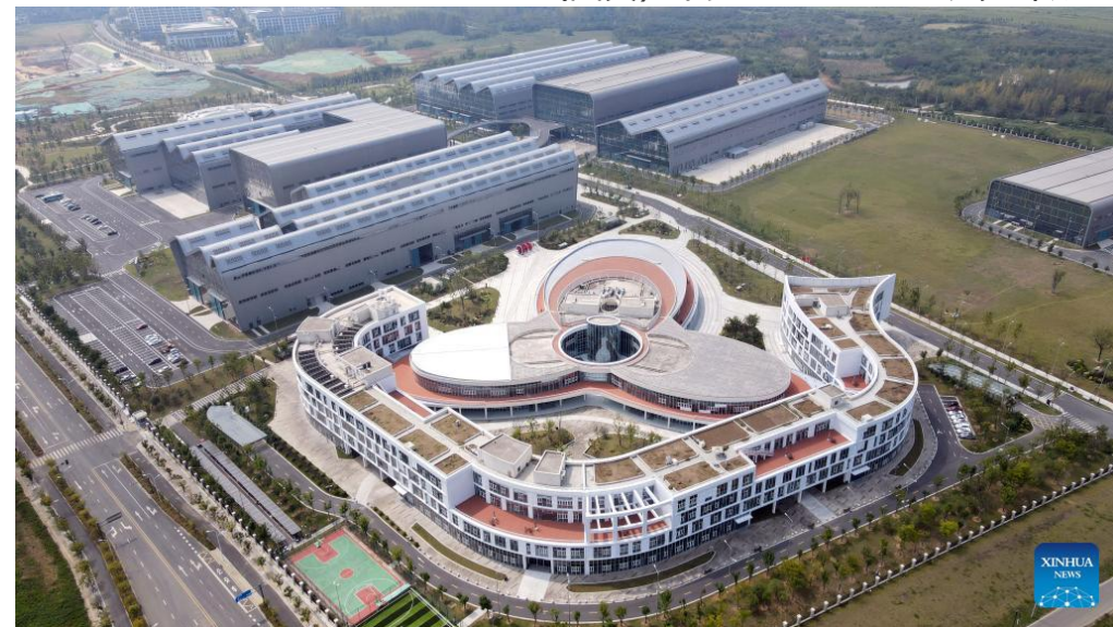
Comprehensive Research Facility for Fusion Technology (CRAFT) in Hefei, east China's Anhui Province
