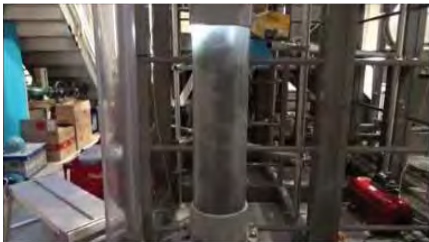
Inside of Pipe
