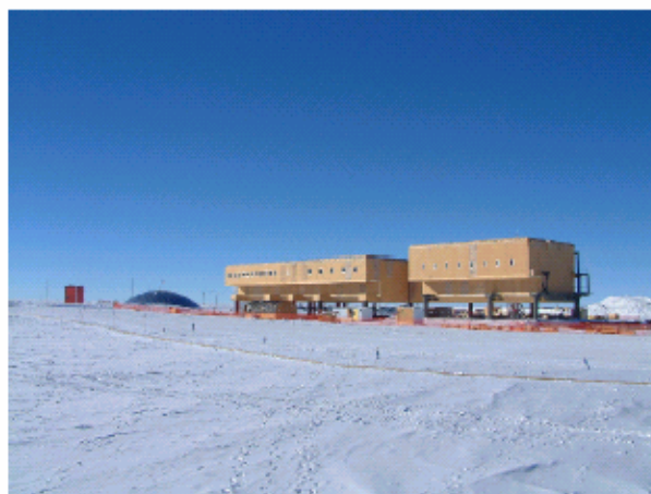
The isolated South Pole Station, currently under construction in Antarctica.
