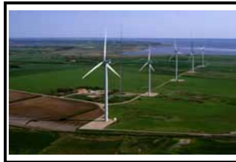
Wind Power Generation
