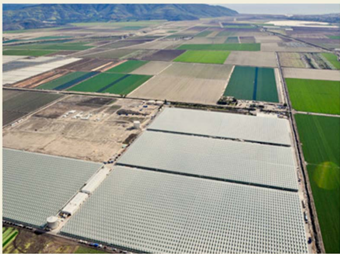
PRE-EXPANSION AERIAL VIEW CAMARILLO, CA
