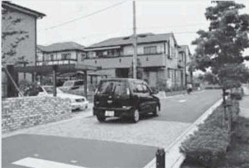
Speed bump in residential area
