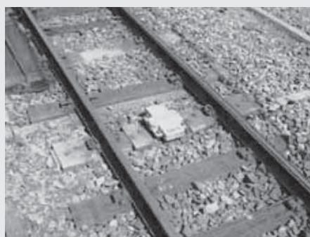
Automatic train stop (ATS) device
