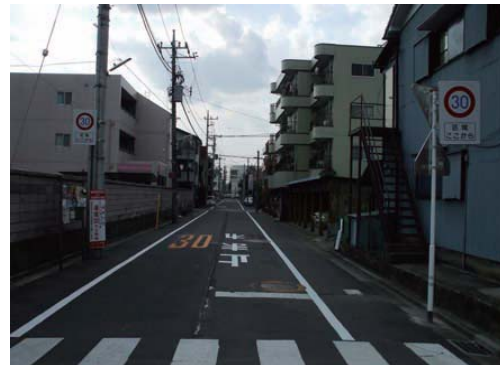
After the measures (the center line erased, side strips installed, area regulations sign on a backboard installed)
