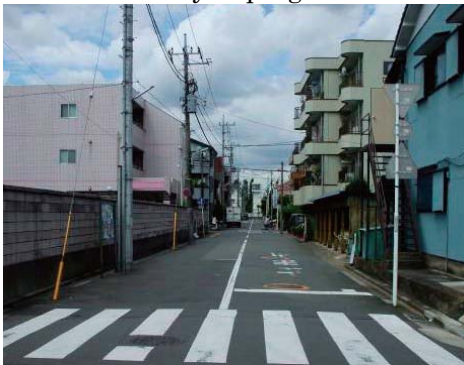
Before the measures (with the center line)
