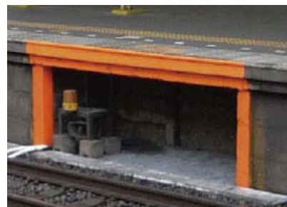
Evacuation space under a platform
