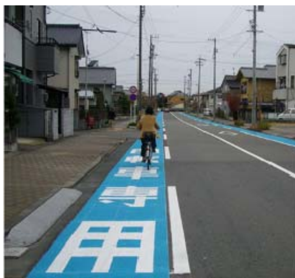
Installation of bicycle lanes (Kikugawa, Shizuoka Prefecture)
