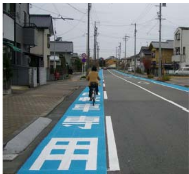
Installation of bicycle lanes (Kikugawa, Shizuoka Prefecture)
