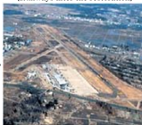
[Runways after the restoration]
