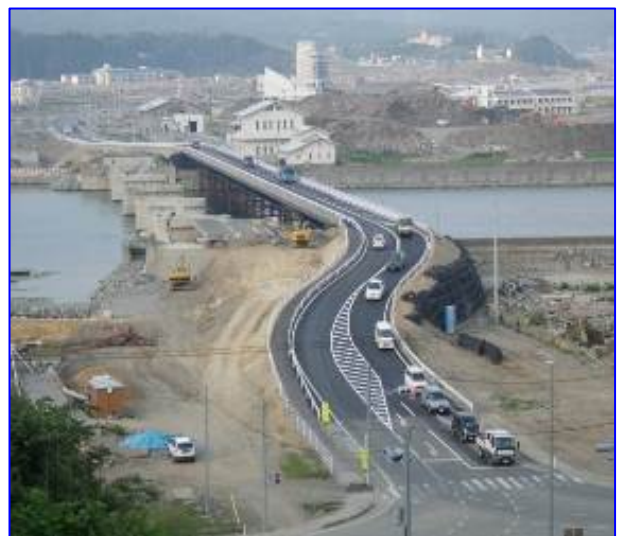
(The temporary bridge after its opening)
