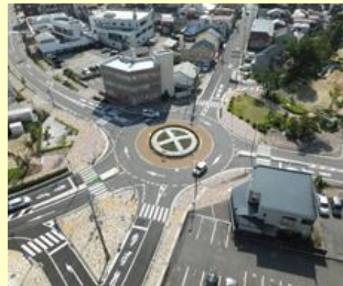
Planar intersection structure of roundabout (Towacho Roundabout, Iida City, Nagano Prefecture)
