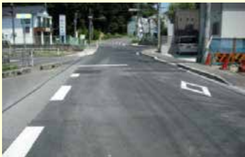
Before execution of the measures
