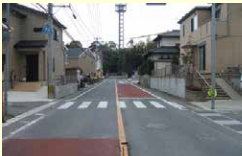
Before execution of the measures
