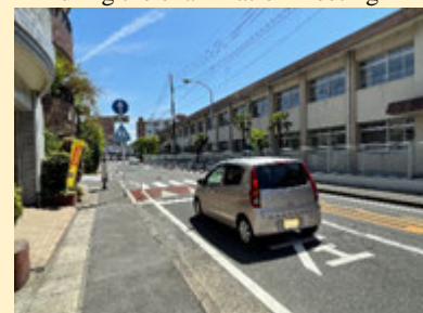
Appearance of slightly raised smooth pedestrian crossings after installation
