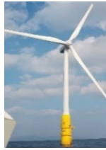
Floating type offshore wind power turbine (in the offing of Goto city, Nagasaki prefecture)
