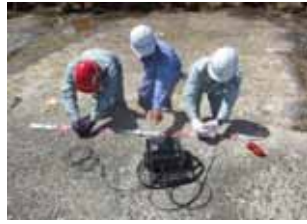
護岸の点検・補修
