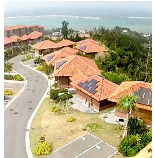
DC-power-transmission network system installed at the teacher lodgings of OIST
