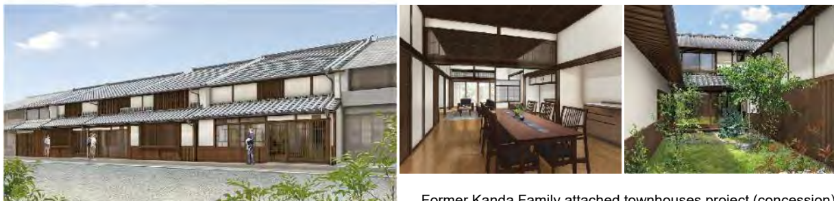
Former Kanda Family attached townhouses project (concession) (Tsuayama, Okayama)
