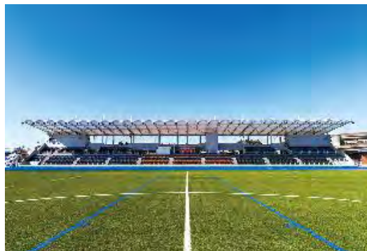
Yanagishima sports park development project (Chigasaki, Kanagawa)
