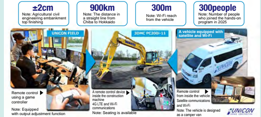
Integration of 3DMC backhoe, remote operation technology, and satellite communication technology ©UNICON
