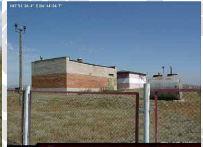
F. Hatch and tank
